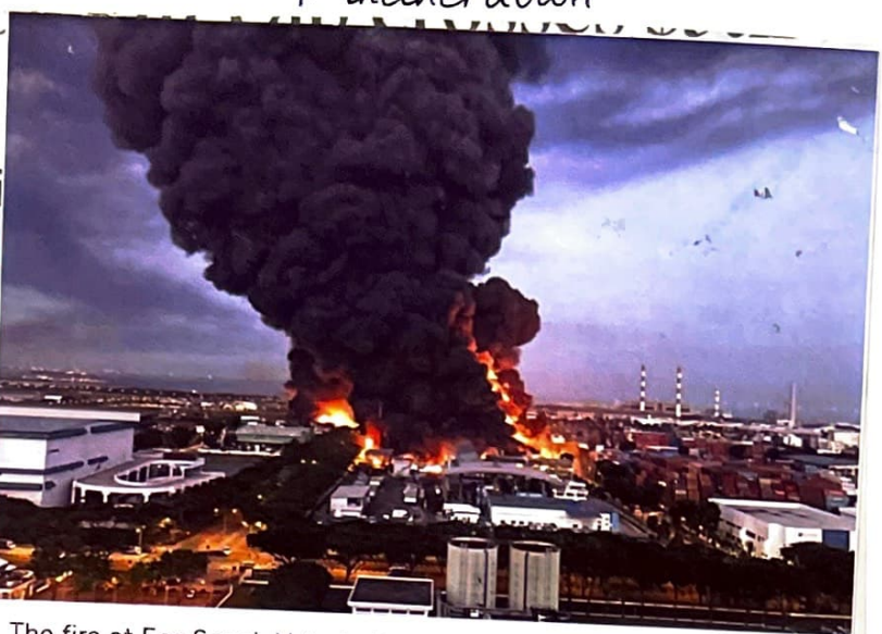
The fire at Eco Special Waste Management's Tuas plant on Feb 23, 2017. It broke out when a worker was discharging recovered liquid hexane from a product tank into a plastic intermediate bulk
